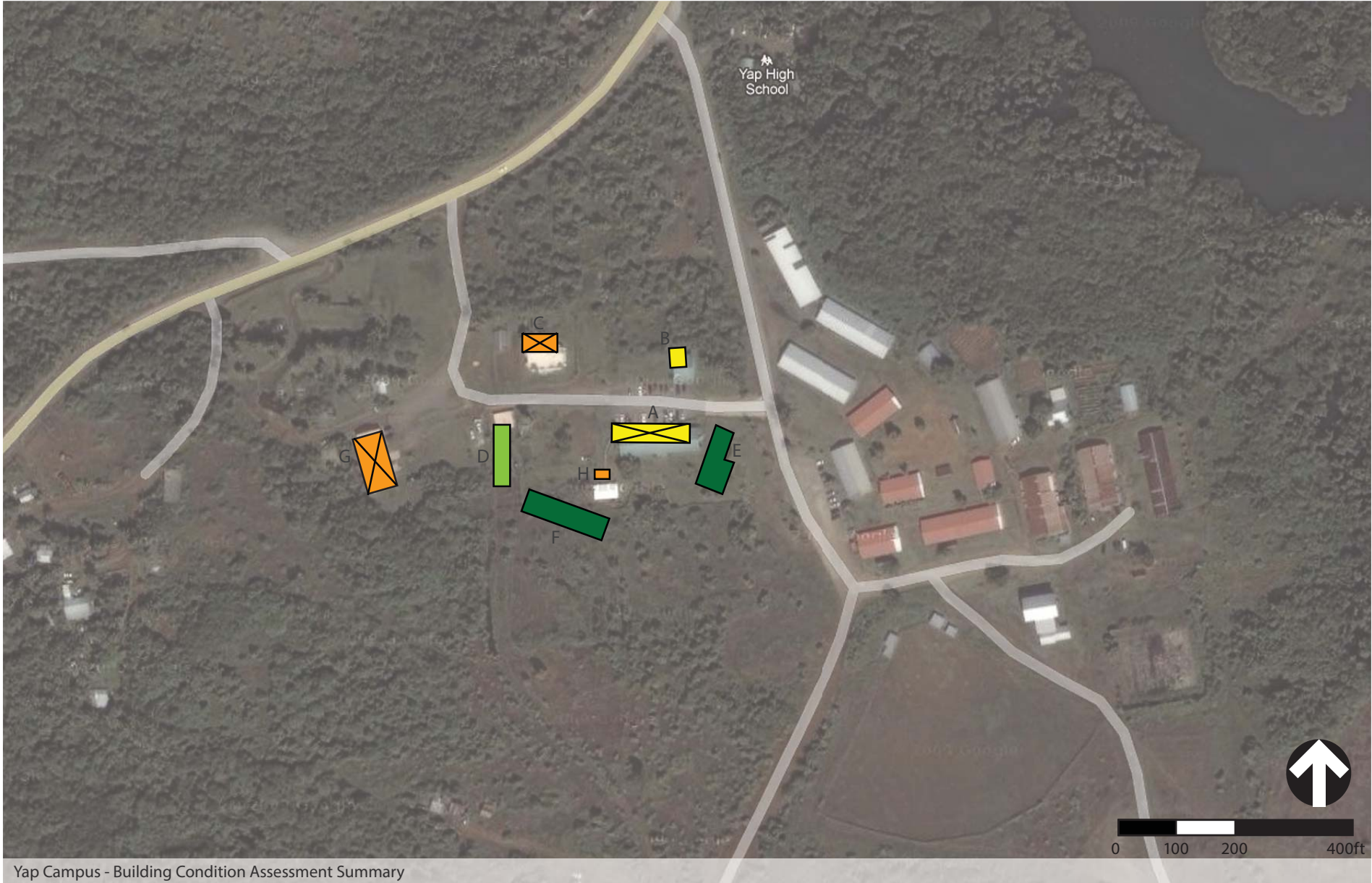
Yap Campus - Building Condition Assessment Summary
