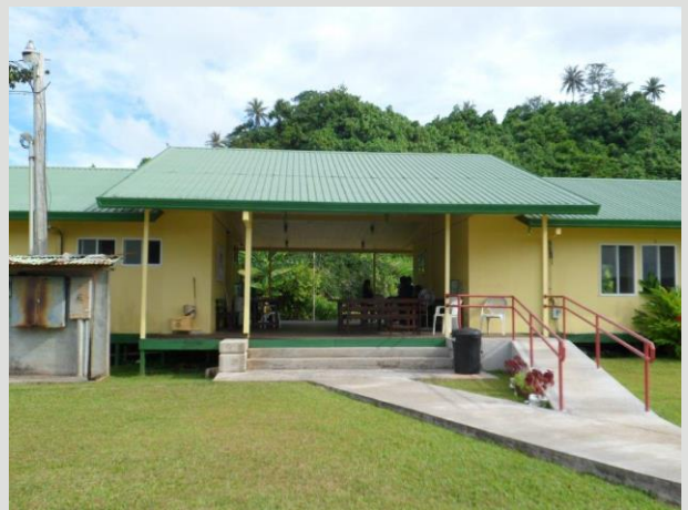
Raised and covered area in the centre of the administration block
