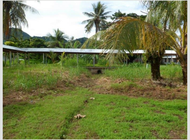
Drainage and culvert through the centre of the site
