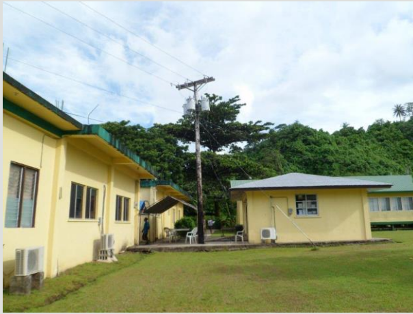
Power lines crossing through the middle of the campus
