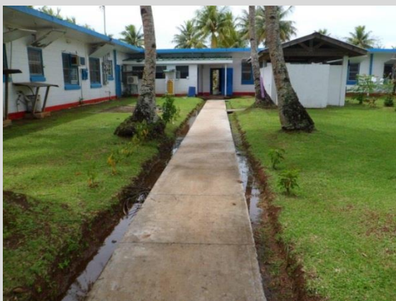
Drainage issues around the northern residential courtyard
