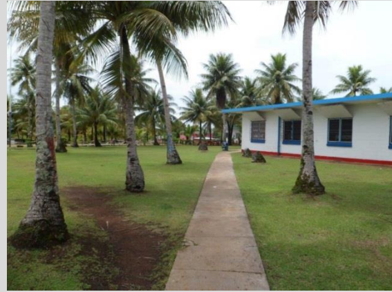
Informal path being formed to the security post - provide a formed walkway
