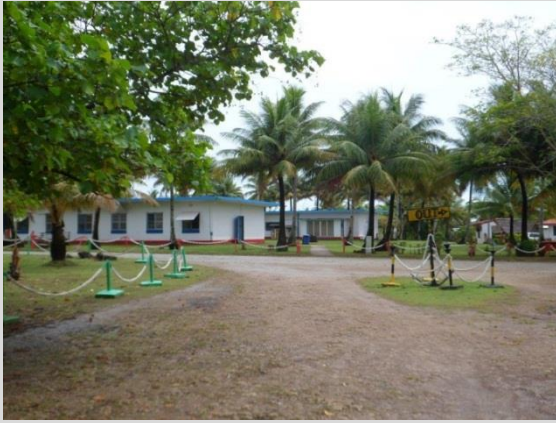
View across the road looking towards the southern wing of the male living quarters. Provide a formed walkway and rain shelter between both sides of the campus
