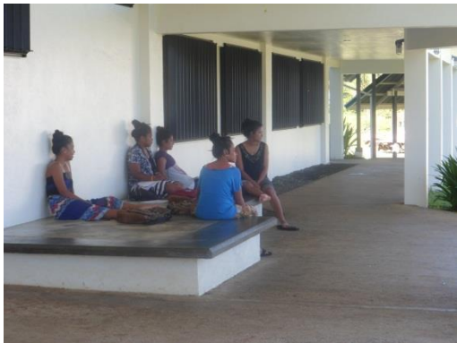
Figure 5: Stone slab seating at the entrance to the Learning Resource Center at the National campus
