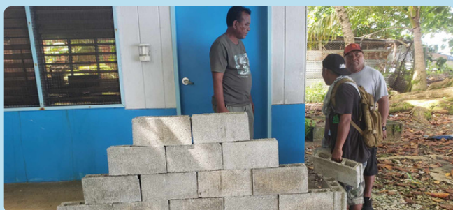
Building a masonry structure.
