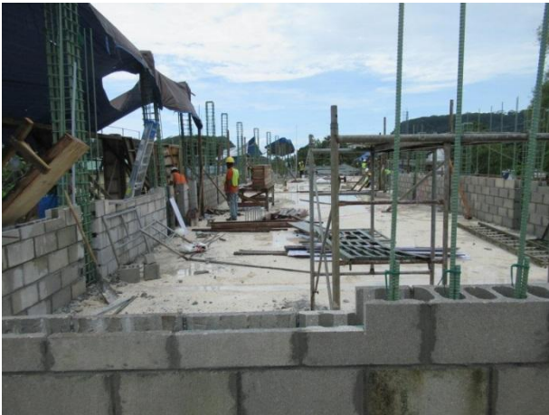
Construction of Walls on the second floor in progress
