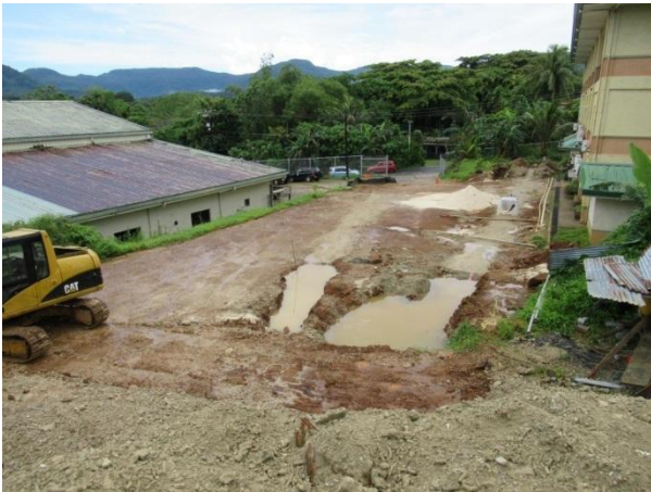
Centralizing Electrical Distribution System
